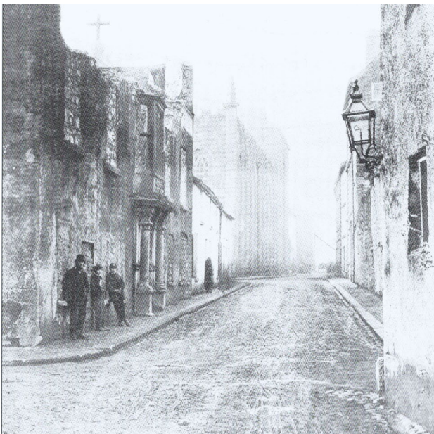
The derelict Browne mansion ‘in a derelict town’ and the well-known Browne doorway at the corner of Lower Abbeygate Street and St Augustine Street c. 1904. From Archaeological Investigations in Galway City 1987-1998 .
