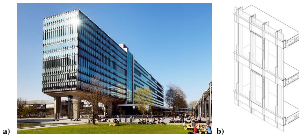
Figure 1: a) Atlas building at TU/e, photo by Bart van Overbeeke, (TU/e, 2019). b) Atlas façade design with parallel openable windows (Arch Daily, 2019).
